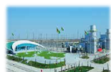
Water Plant | Turkmenistan 1 x 2500 kVA
