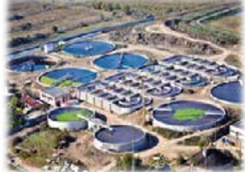
Halac Water Purification Plant | Turkmenistan 2 x 1125 kVA
