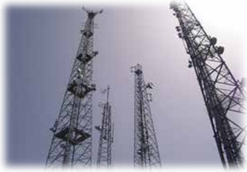
Telecom Base Stations | Georgia 276 x Several Sized Gensets
