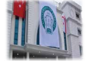
Hospital of University of Kyneria | Cyprus 1 x 440 kVA
