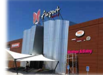
Airport Mall | Cyprus 3 x 700 kVA (Synchronized)
