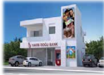
Near East Bank | Cyprus 11 x Several Sized Gensets
